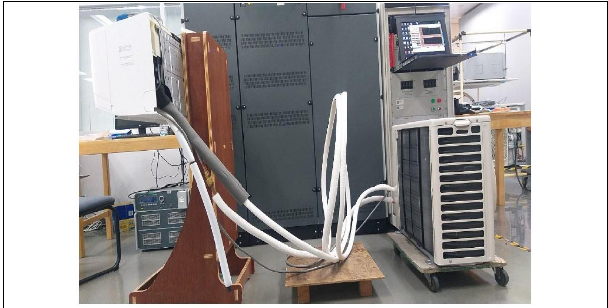
Figure AIII.3: Harmonic current emission, Voltage fluctuation and flicker test set-up
